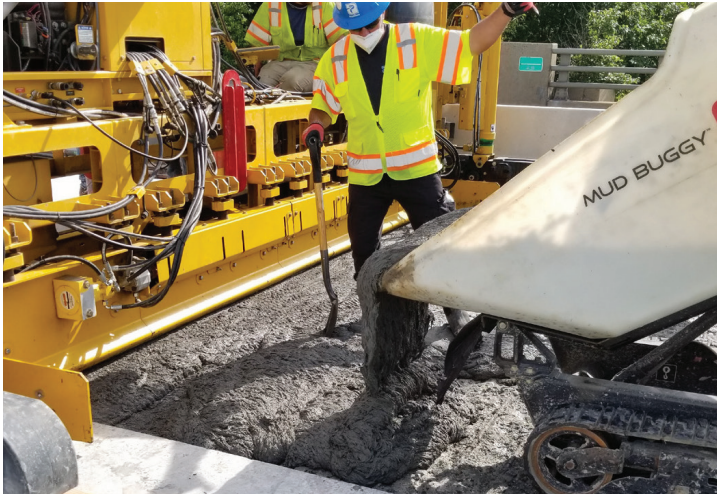
Ductal material being transported and placed with a specialized UHPC paver
