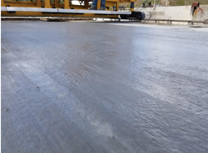
Ductal Overlay surface finish following placement with a paver
